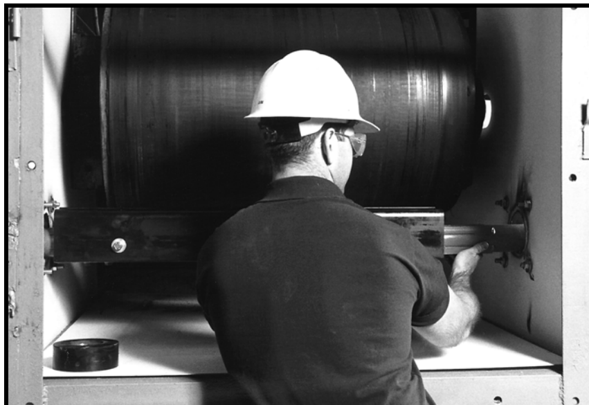
Figure 4. Installing belt cleaner mainframe
